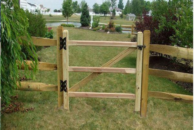
Split Rail Gate Style Example
